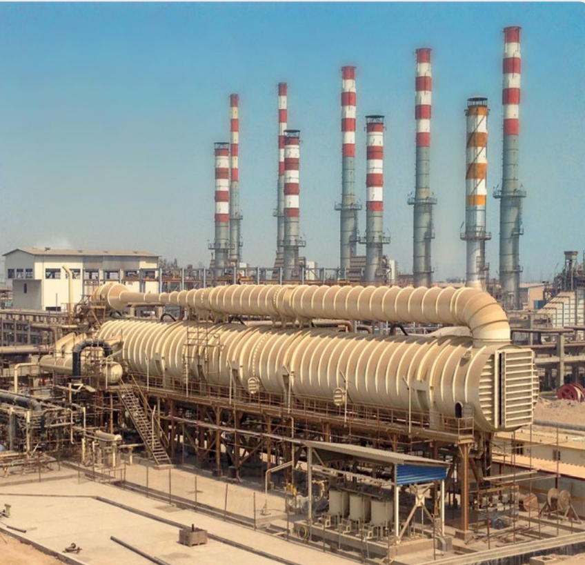
Process of Desalination: Boiling and cooling the steam to make potable water.
